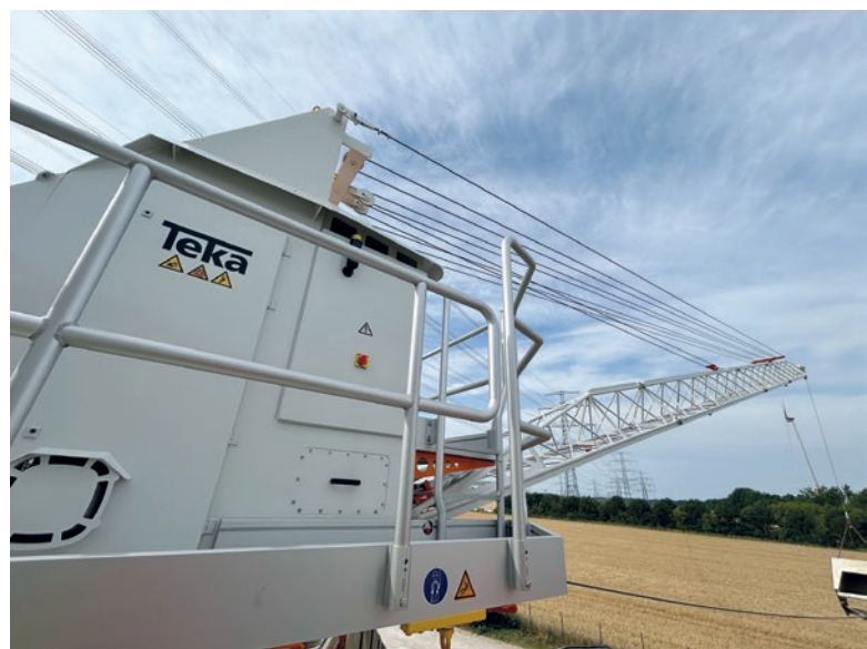
The main control cabinet with integrated air conditioning unit is attached directly to the scraper.
