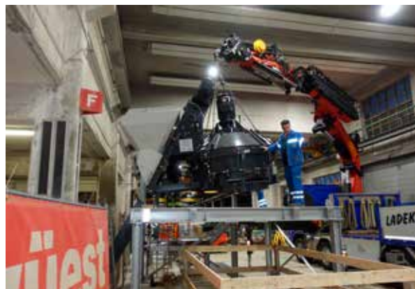
The new Teka turbine mixer was installed in January 2019
