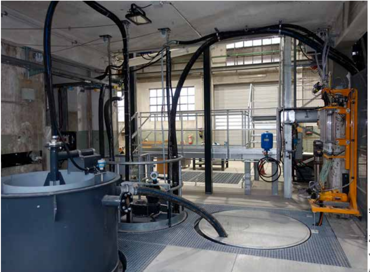
A Hölscher Klärfix water recycling unit was installed
