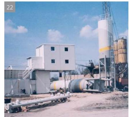
18-22 | Erection of MIXOMAT THZ 3000 C 1-R with heavy duty TEKA pan-type mixer with separate mixer and weighing scale platforms and complete housing for the plant.
