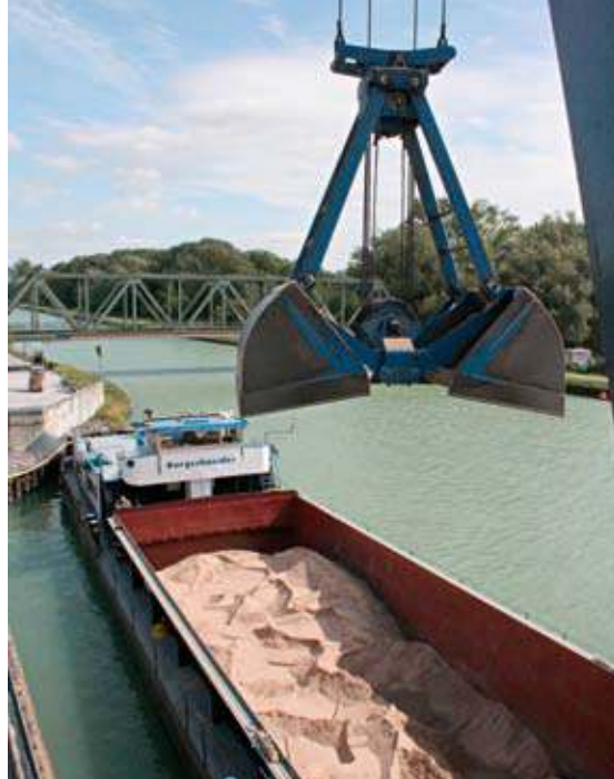
Fig. 2 a+b Aggregates arrive at pebüso by ship and are transported by crane to the twelve new silos.
