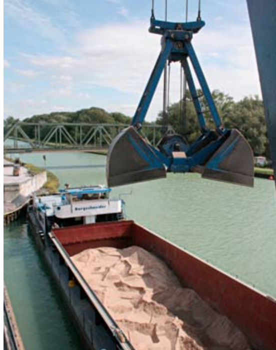
Fig. 2 a+b Aggregates arrive at pebüso by ship and are transported by crane to the twelve new silos.
